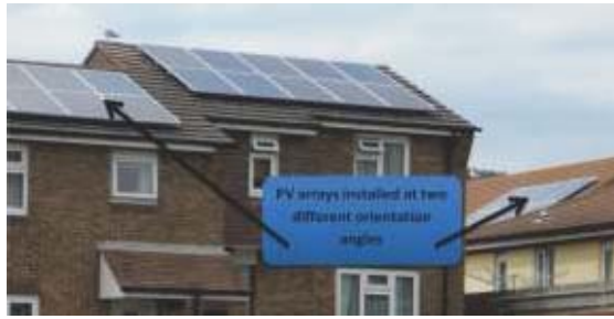
Figure 1: PV arrays at different orientation angles in Brighton, UK – photo taken during July 2015 by the researcher
