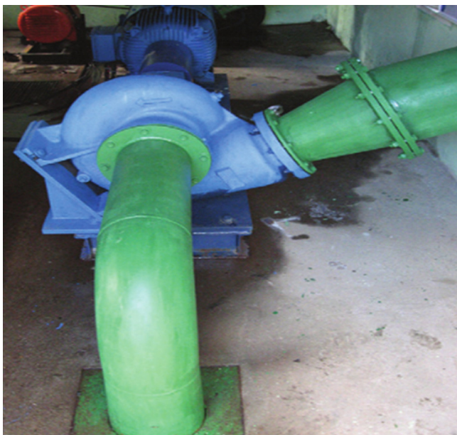
Fig. 2. Installed pump as turbine [23].
