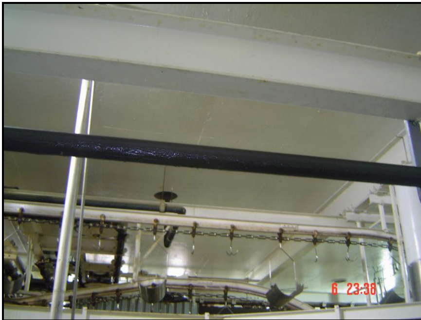
Figure 2.4: Underside of a parapet roof/ceiling
