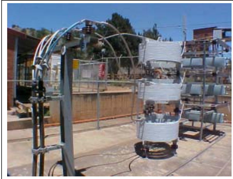
Fig. 1.1. ABB Powertech harmonic filter bank.
