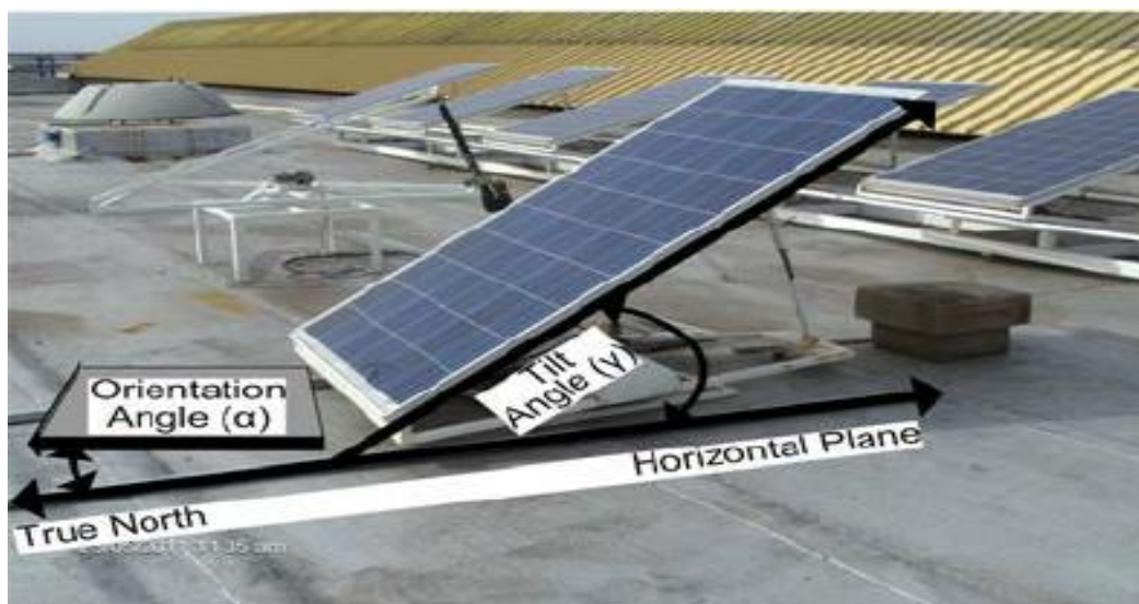
Figure 2.9. PV module showing orientation ( \gamma ) and tilt ( \alpha ) angles (Asowata et al. , 2012).
