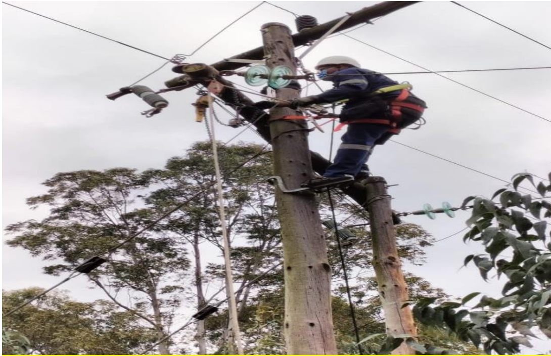
Figure 15: Worker performing a task while working at heights
