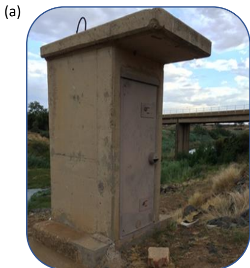
Figure 3.16: Gauge station at (a) Krugersdrift and (b) Bultfontein station
