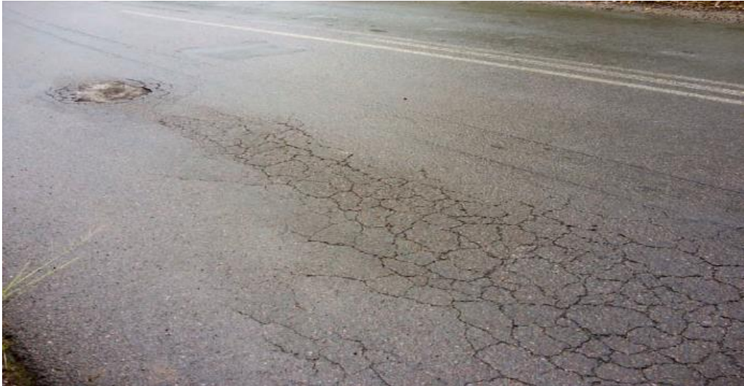
Figure 2.8: Cracking because of support failure
