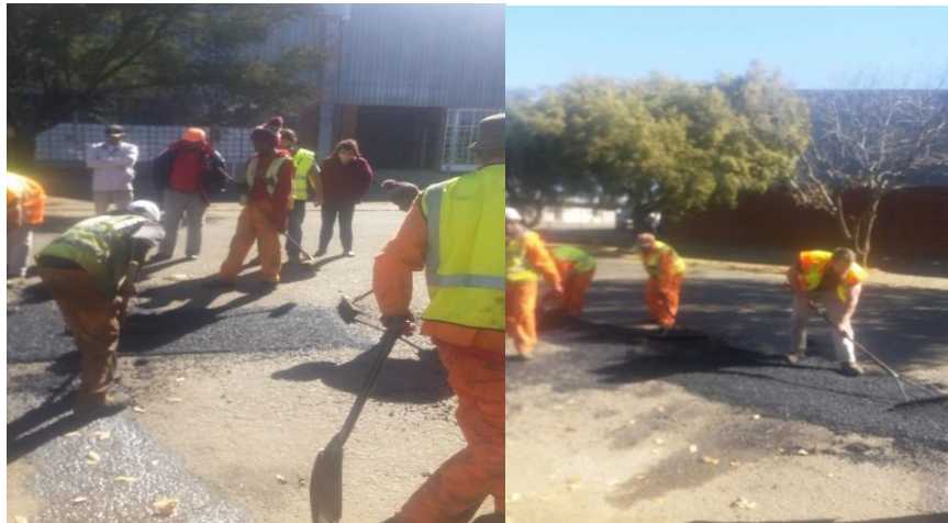
Figure 5.1: Pothole repairs in Motheo District
