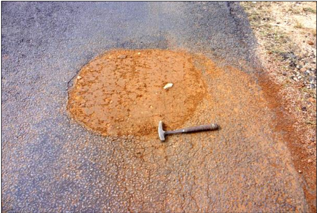
Figure 2.9: Poor Pothole Maintenance
