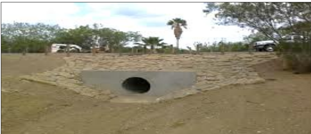
Figure 2.5: Culvert to drain storm water from a road network
