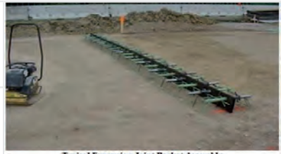
Typical Expansion Joint Basket Assembly
