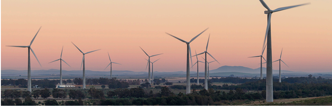
Figure 3: Gouda Wind Farm Outside Cape Town [21]
