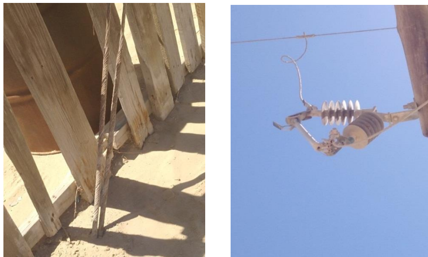
Figure 4.6: a) Corrosion on the stay on one of the poles, b) Corrosion on one of the newly installed jumpers
