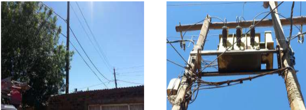
Figure 4.9: a) MV and LV lines connected to the same poles, b) An overloaded transformer
