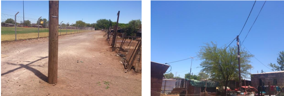
Figure 4.11: a) A pole in the middle of a street, b) Tree underneath the line
