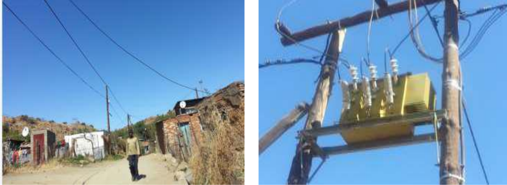
Figure 4.8: a) Low hanging concentric cables in Kuyasa, b) Pole-mounted transformer installed without MV Fuses on the primary side
