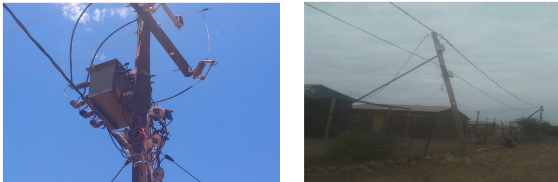
Figure 4.12: a) A pole-mounted transformer with oil leaks, b) One of the leaning LV poles in Newtown
