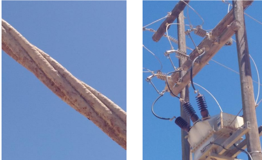
Figure 4.5: a) Corrosion on the conductors, b) Ageing and corroded breaker
