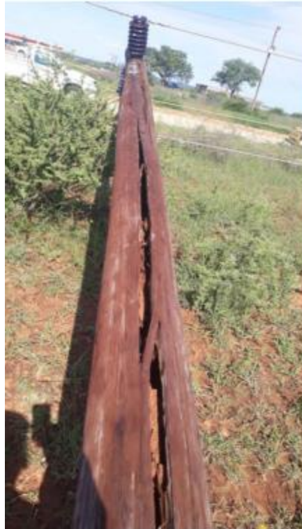
Figure 2.7: Broken utility wood pole [49]
