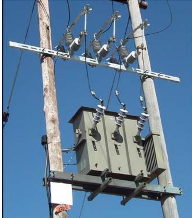
Figure 2.3: An example of a pole-mounted transformer [42]
