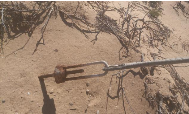
Fig .7. Stay which is affected by Rust in Sizamile.
