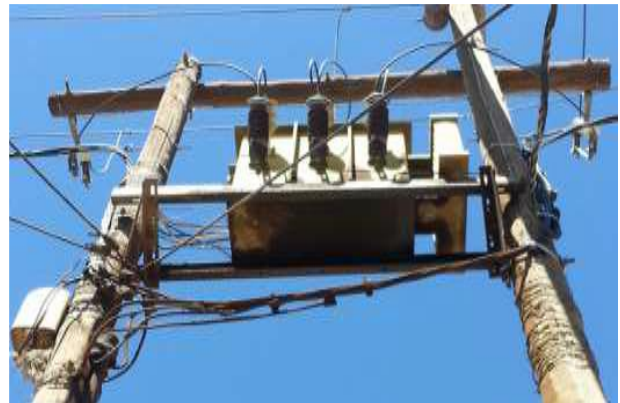
Fig .10. Leaking Pole Mount Transformer due to Overloading
