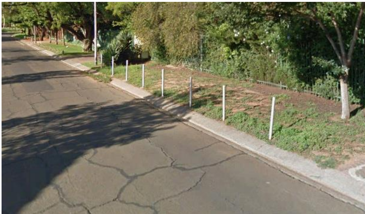
Figure 5-1: Obstructed Sidewalk Network (Google Earth, Accessed in 2017)
