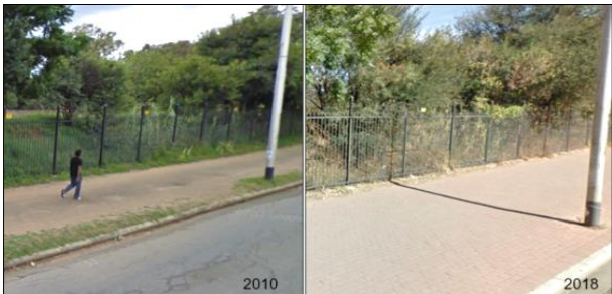
Figure 3-13: Historical imagery from Google Maps Street View showing the sidewalk upgrade in Henry Street, Bloemfontein (Google LLC, 2017).
