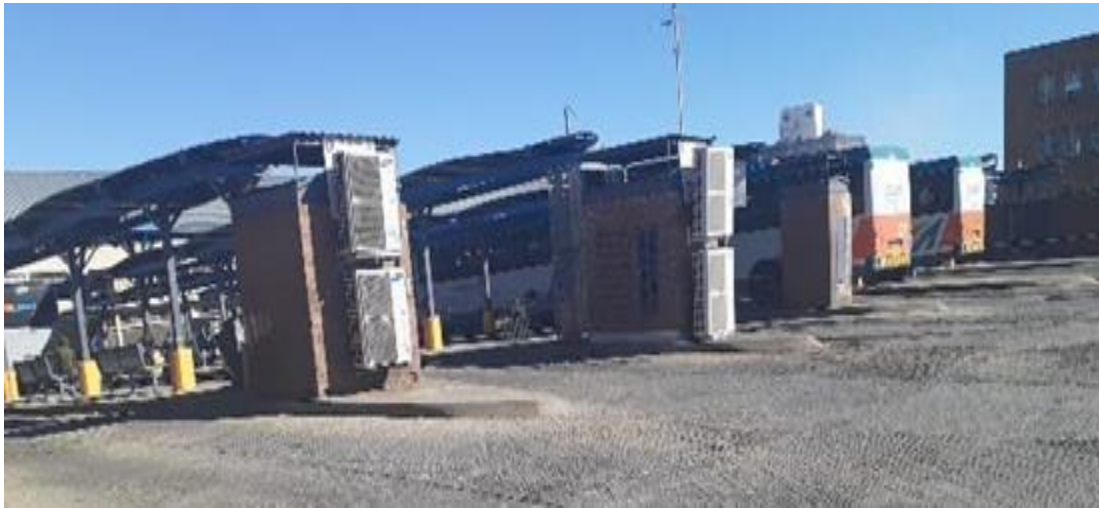
Figure 3. 3: Interstate Busline terminal parking lots and passengers' waiting areas
