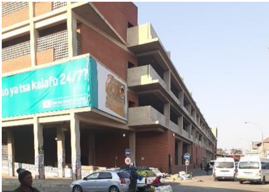
Figure 3. 2: Mangaung Intermodal Transport Facility
