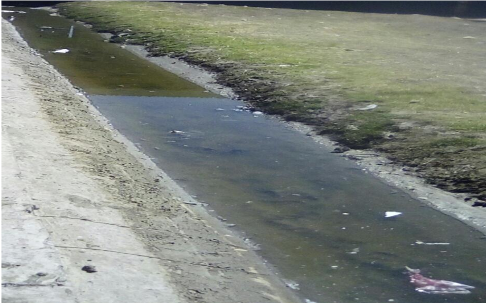
Picture 4.3: Standing water on the school premises
