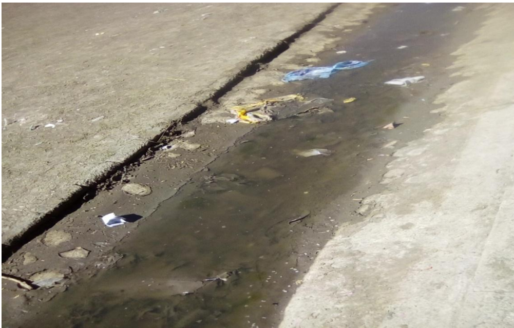
Picture 4.2: A drainage problem
