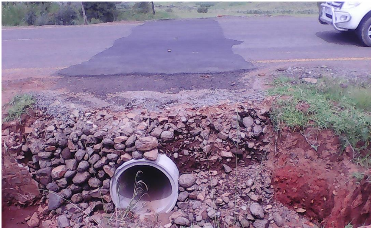
Figure 5.1 Poorly compacted culvert crossing main Sehlabeng road in Maseru.
