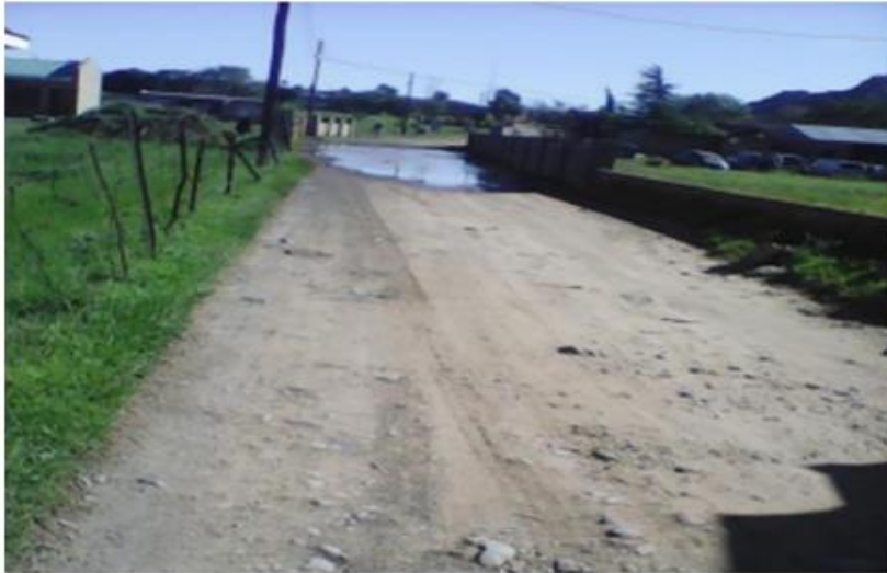
A. Mainly trafficked gravel road leading to Leqele village showing private property projecting into the road and a pool of water in the corridor due to lack of water channels
