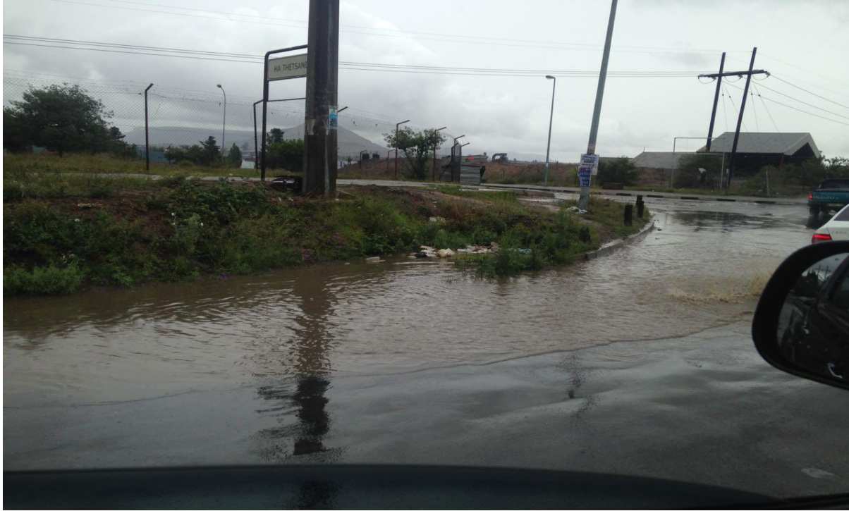
Figure 5.6 Illustrating silted drainages at haThetsane.
