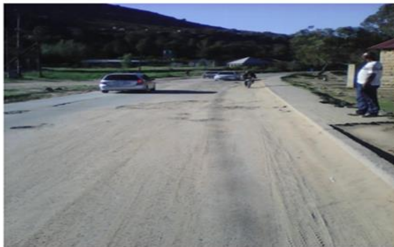
B. Main asphaltic road leading into Qoaling Village showing wearing off pavement layers within 5 years after its construction
