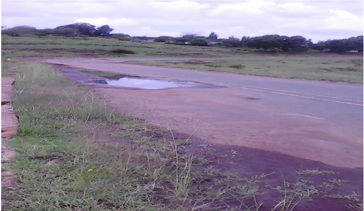
Figure 5.2 Road showing water pond in the carriageway in Sehlabeng Road in Maseru.
