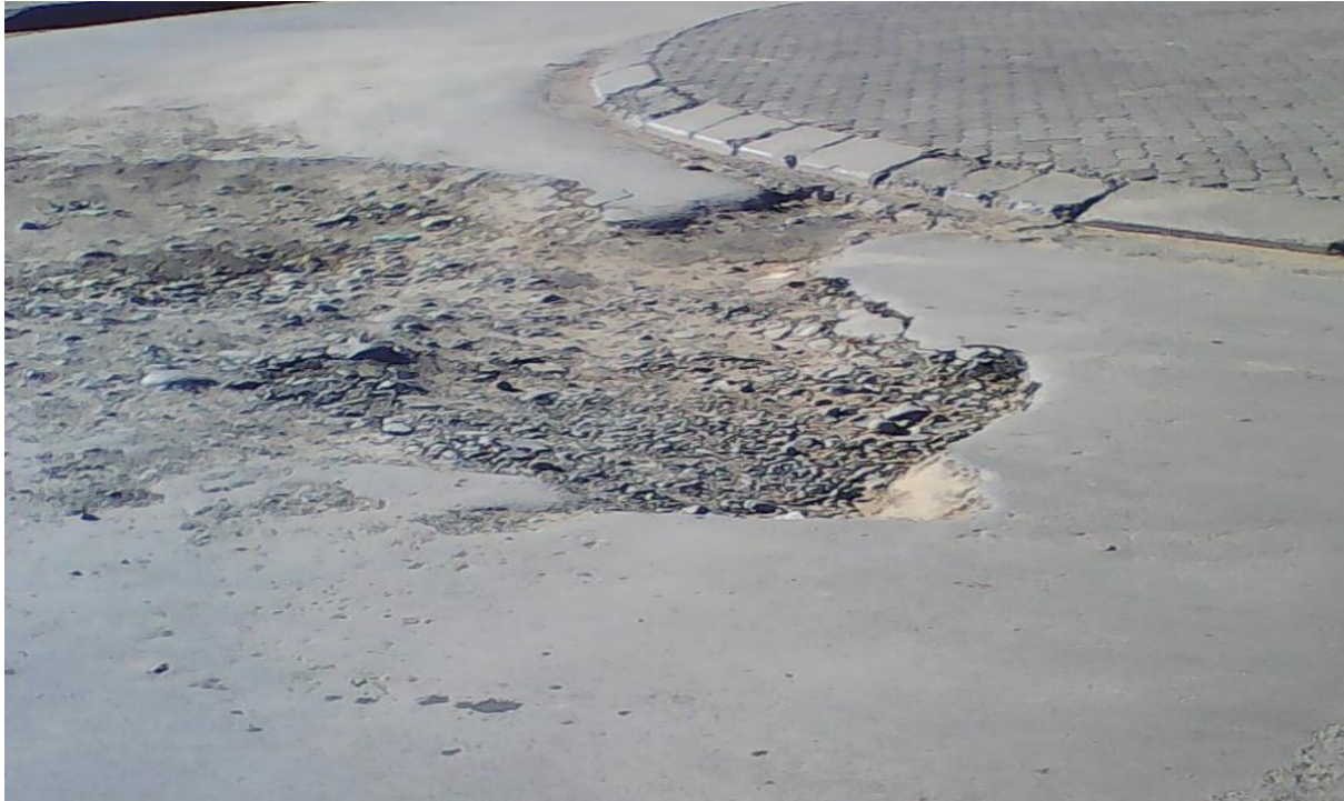
Figure 5.5 Potholes in the traffic control circle Ha Pita.
