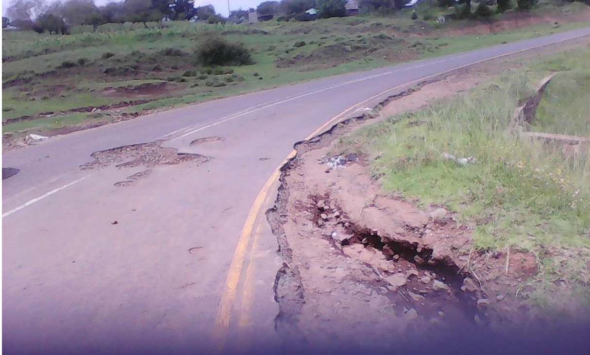
Figure 5.4 shows an inadequate thickness of asphalt layer
