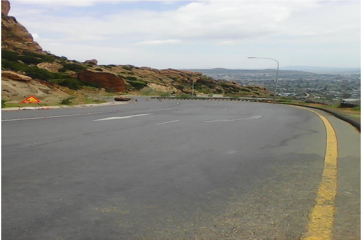
Figure 5.3 A meandering curve with stones protruding into the road carriageway.
