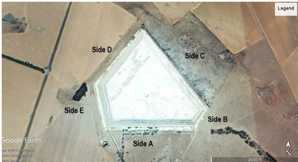
Figure 6.2: Five (5) sides of the tailings dam
