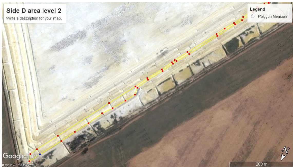
Figure 6.5: Measurements of each segment as polygon area for each of the 5 sides.
