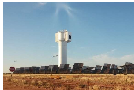
Figure 37 A central tower surrounded by heliostats.
