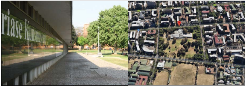
Figure 5. The Pretoria Art Museum (2015) by author, and the location in Pretoria (Google maps 2018)
