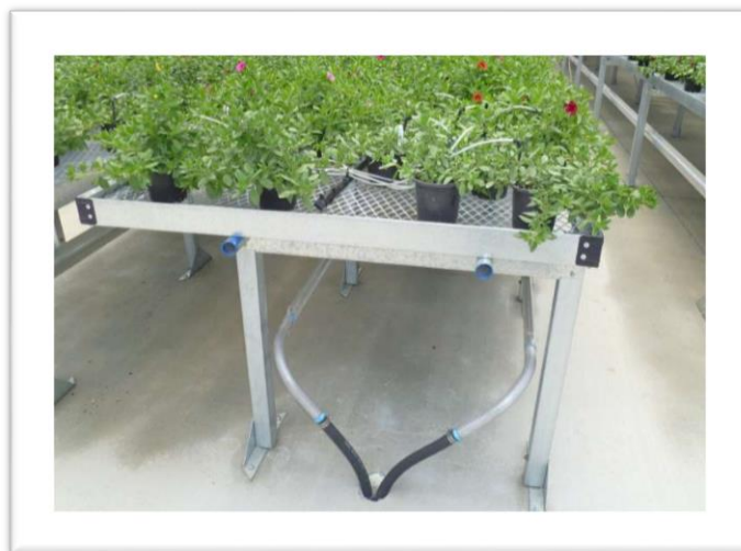
Figure 35 – Under-bench heating system [71].
