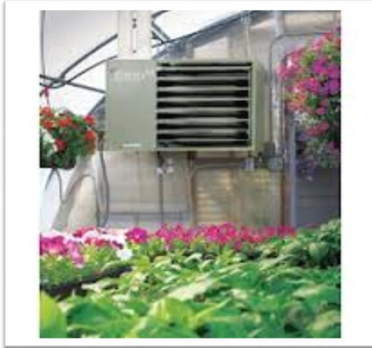
Figure 33 - Unit heater [69].
