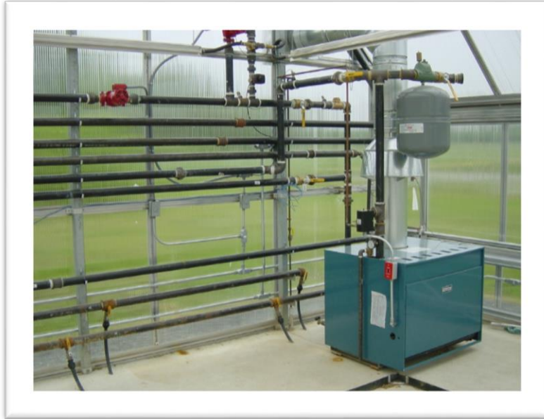
Figure 38 - Perimeter heating system [74].
