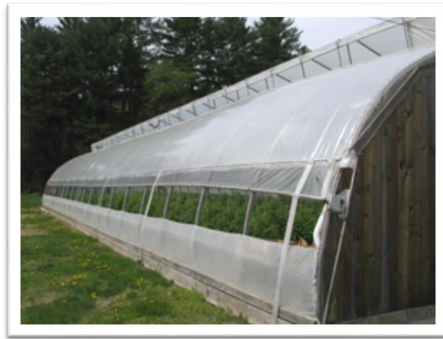
Figure 30 - Roll-up side vent [63].
