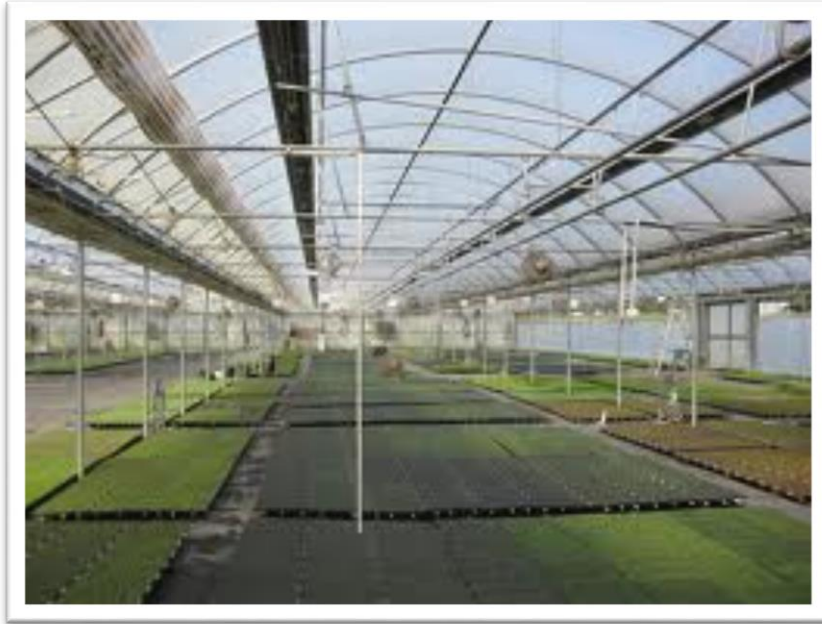
Figure 37 - Overhead heating tubes inside a greenhouse [73].
