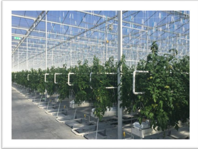
Figure 34 - Pipe/rail heating system [70].
