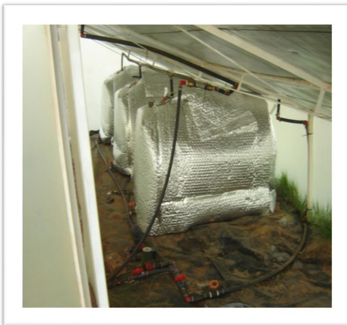
Figure 46 - Hot water storage.
