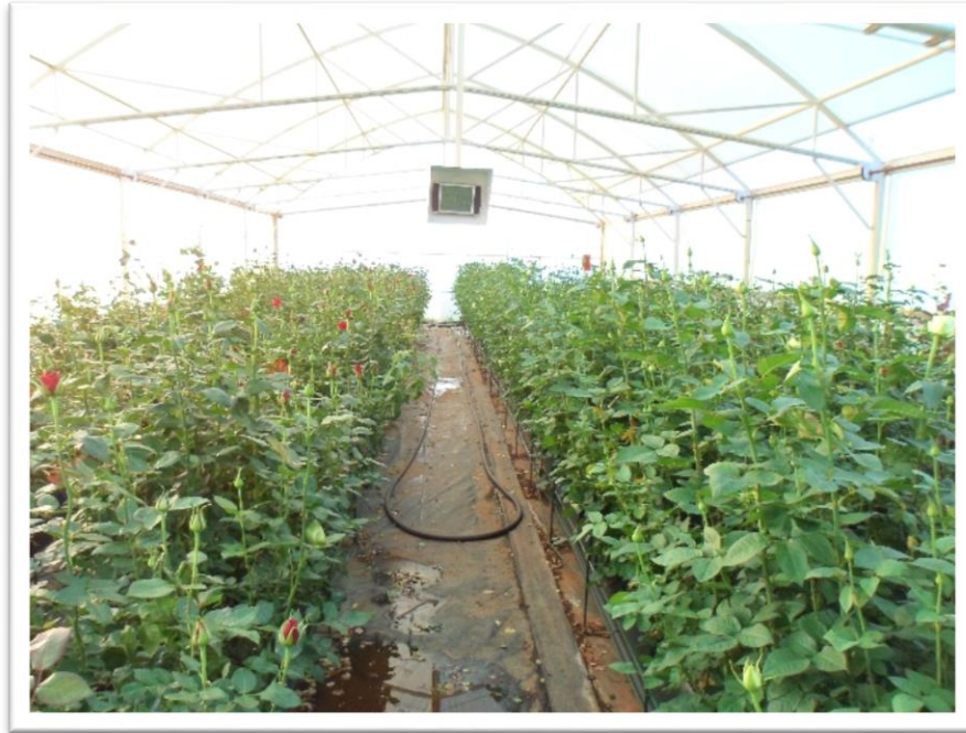
Figure 47 - Heat exchange system installed underneath raised beds.
