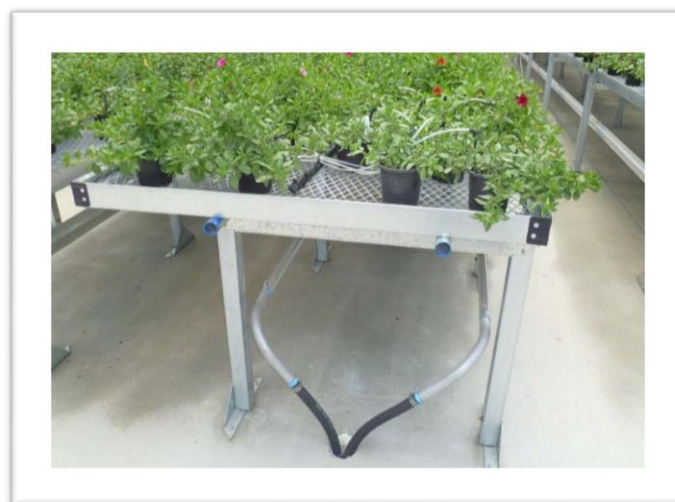
Figure 35 – Under-bench heating system [71].
