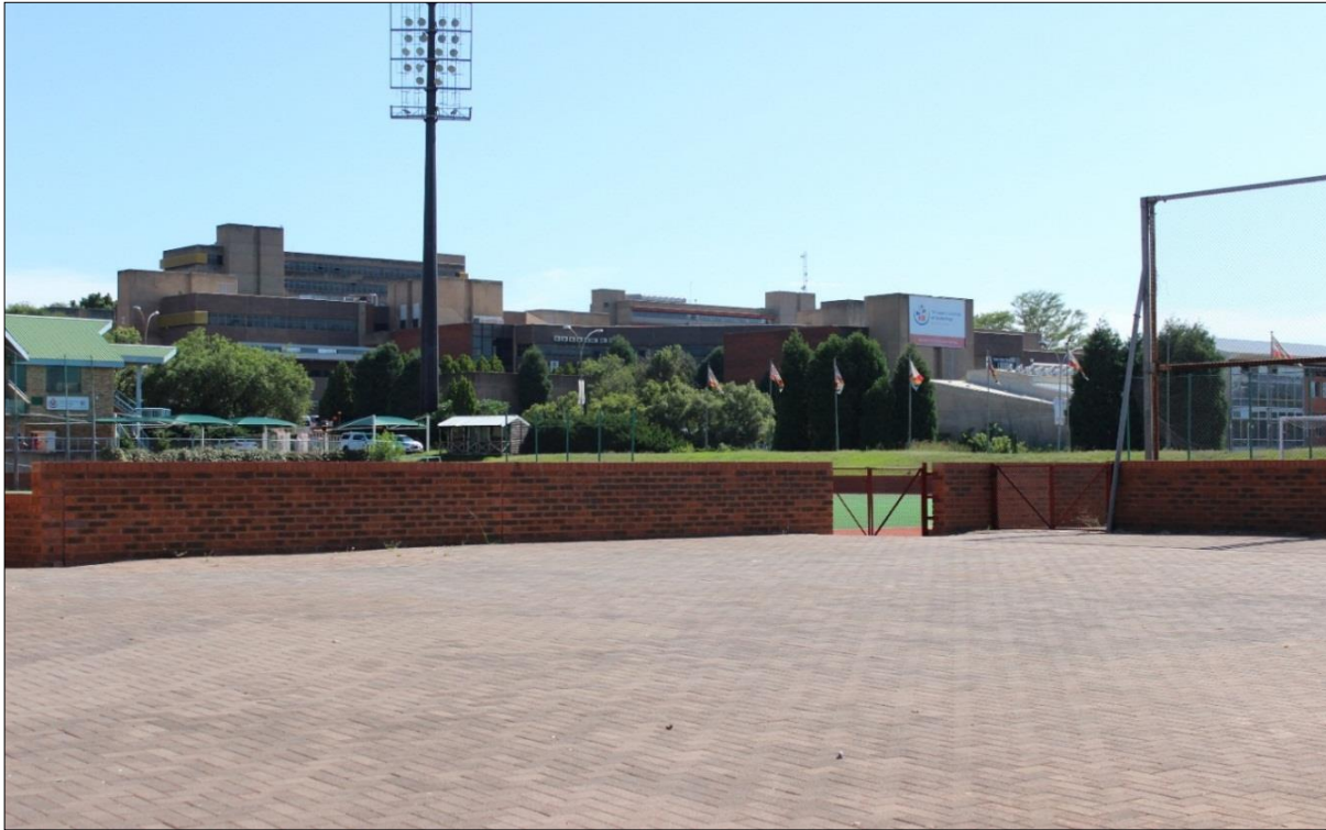
Figure 4.24: Approach views of TUT's Pretoria campus
