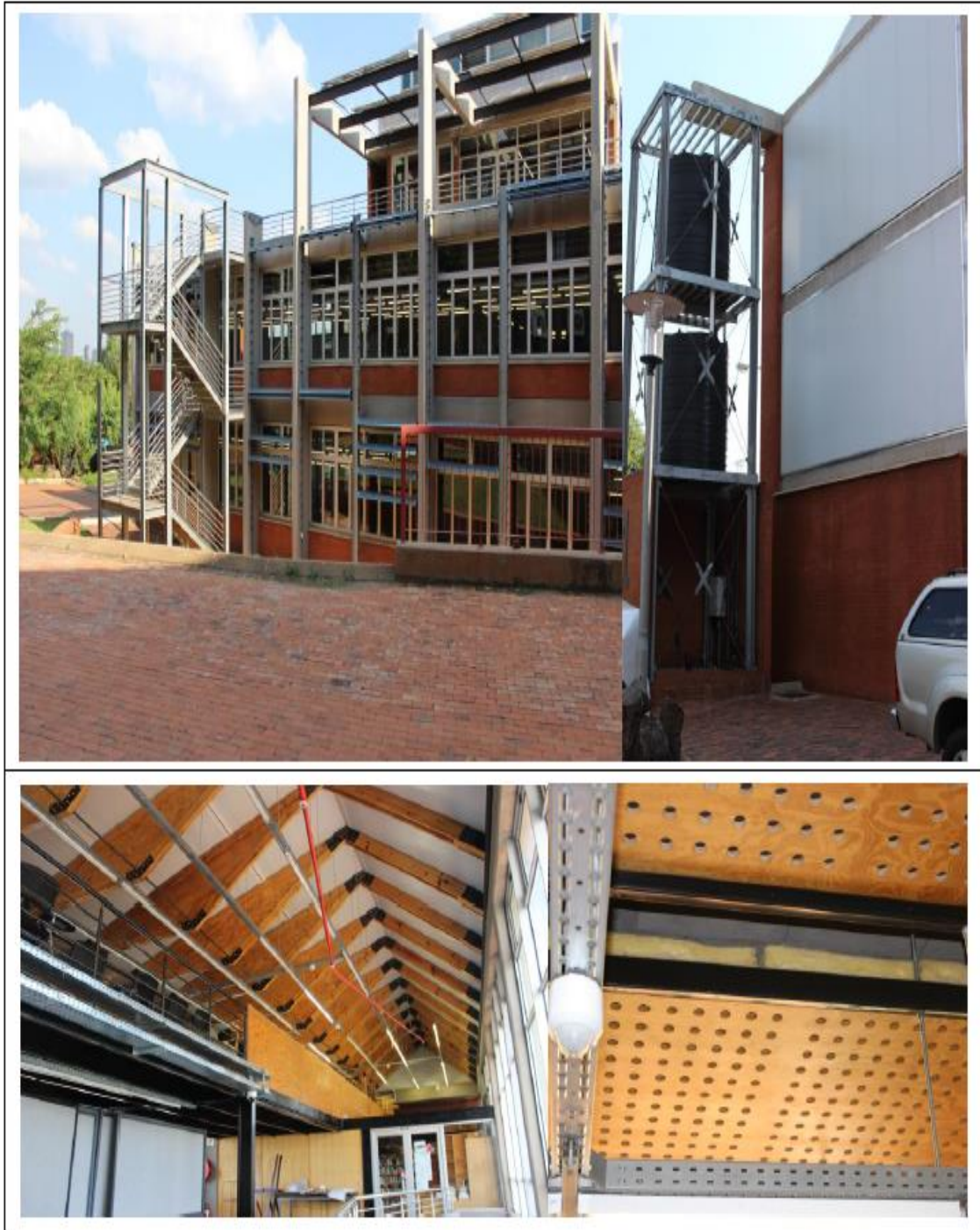
Figure 4.29: Façade features and interior view of building 11
