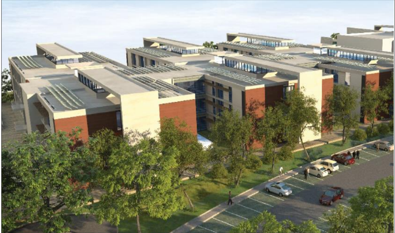
Figure 4.31: DEA building in Pretoria
