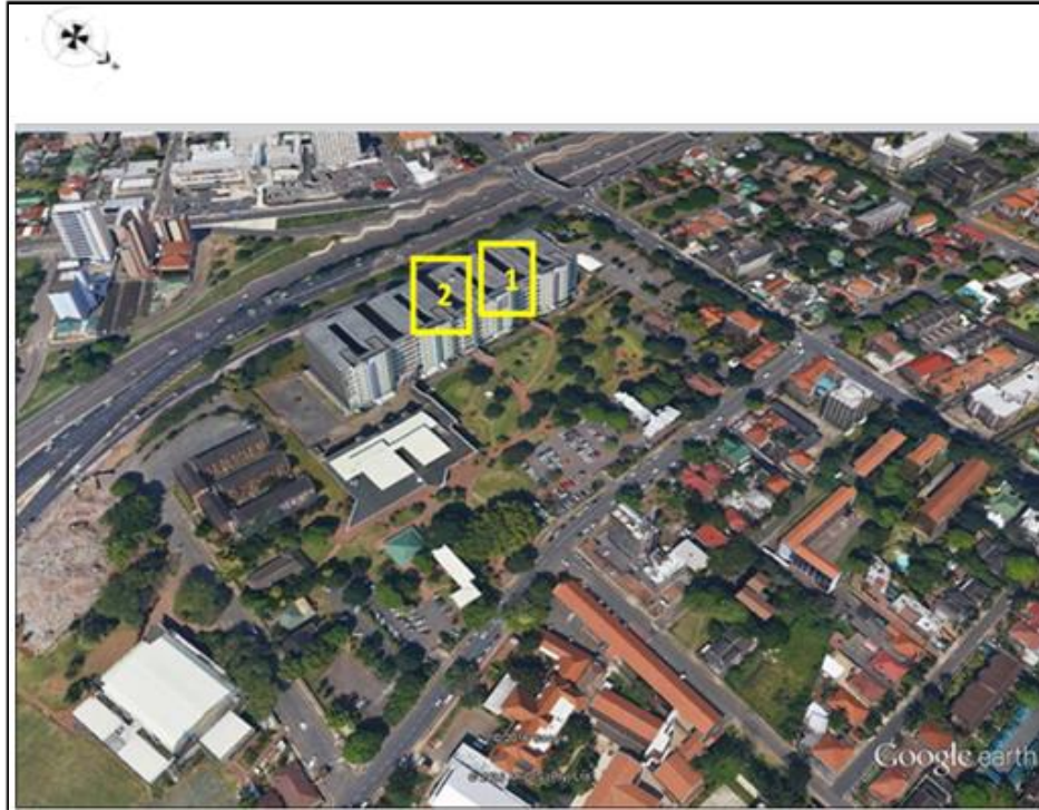
Figure 4.14: Building location and orientation of assessed buildings at Steve Biko campus. 1: S3, 2:S8 Photo: Google earth
