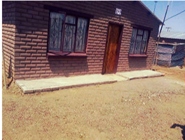
Figure 4-19: Paving in front of the house
