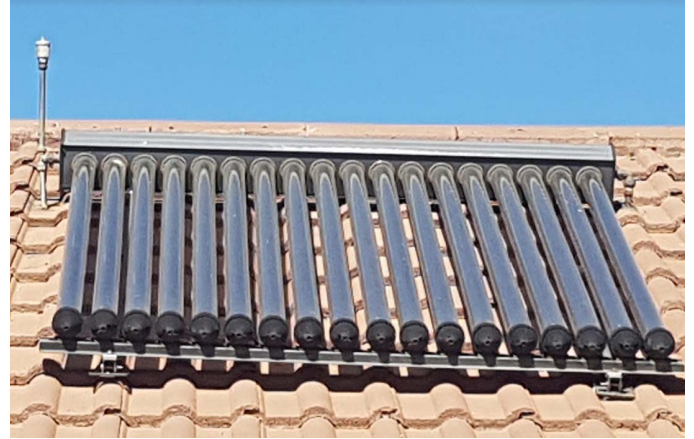
Fig. 1: Solar heat collectors of monitored SWH system
