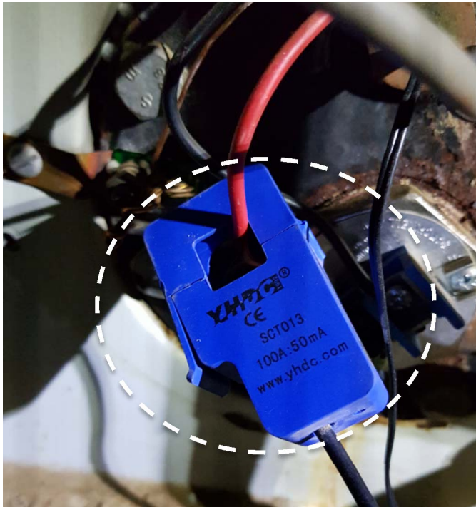
Fig. 3: 100 A CT coupled on the live AC wire to the SWH element
