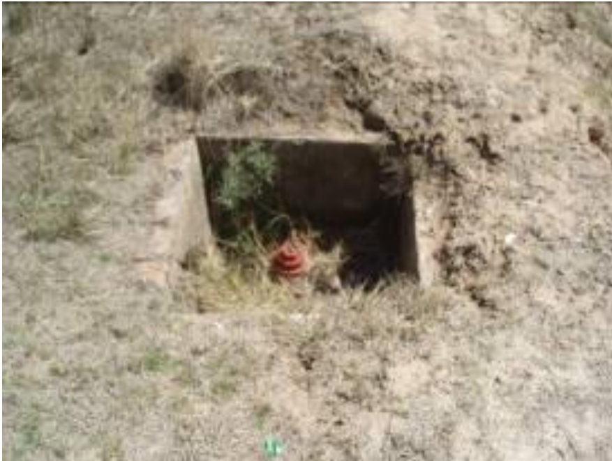
Figure 3.3: Stop valve on top of mine 1
