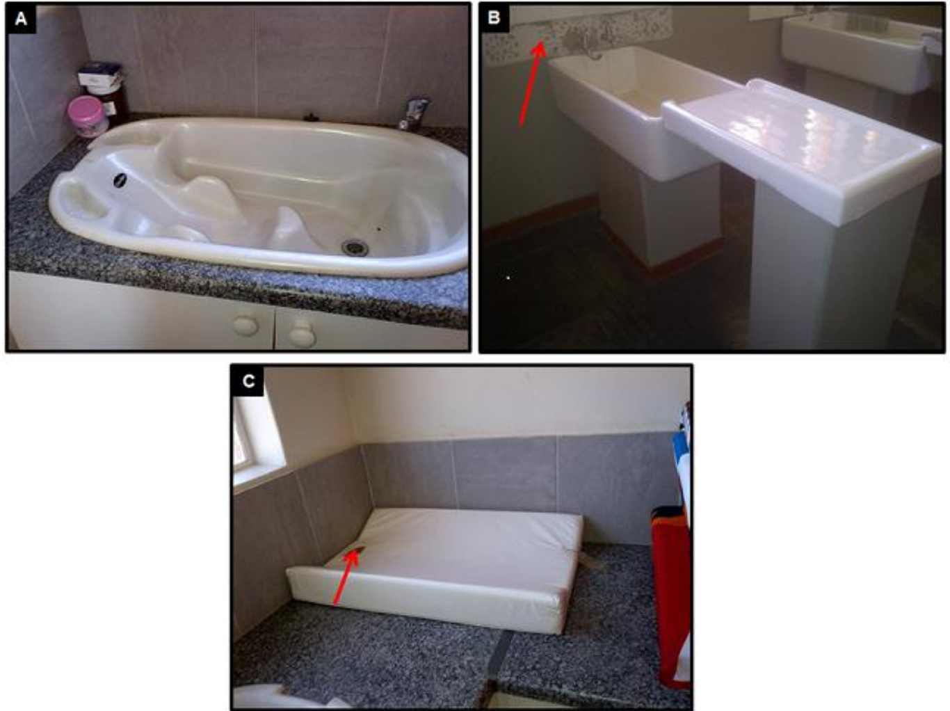
Figure 2.15: A-B Diaper changing stations. A- Diaper changing toddler wash basin; B- Diaper changing wash basin and changing surface; C- Impervious diaper changing mat.
