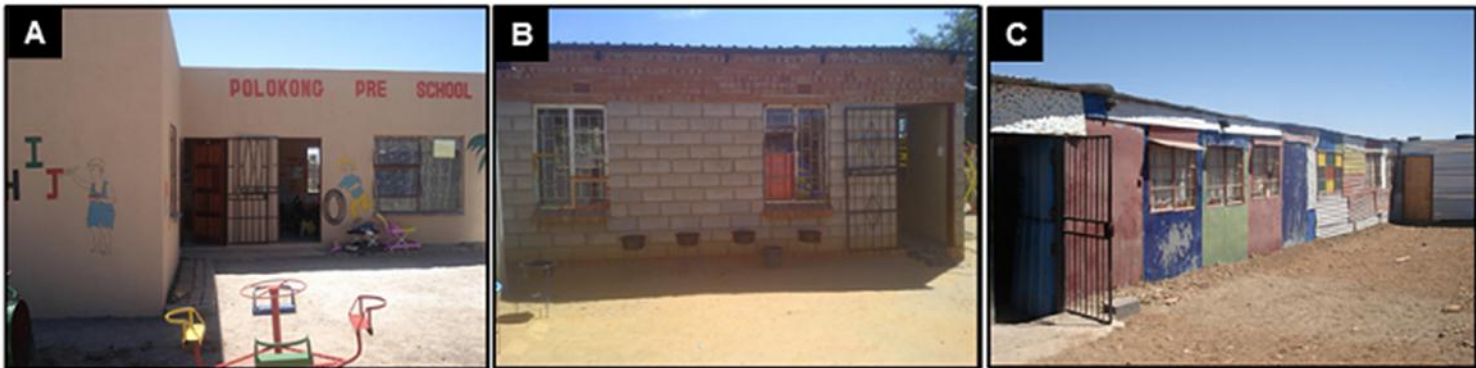
Figure 2.3: A-B indicating the type of childcare facility structures. A and B- Concrete structures; B- Zinc sheeting structure.
