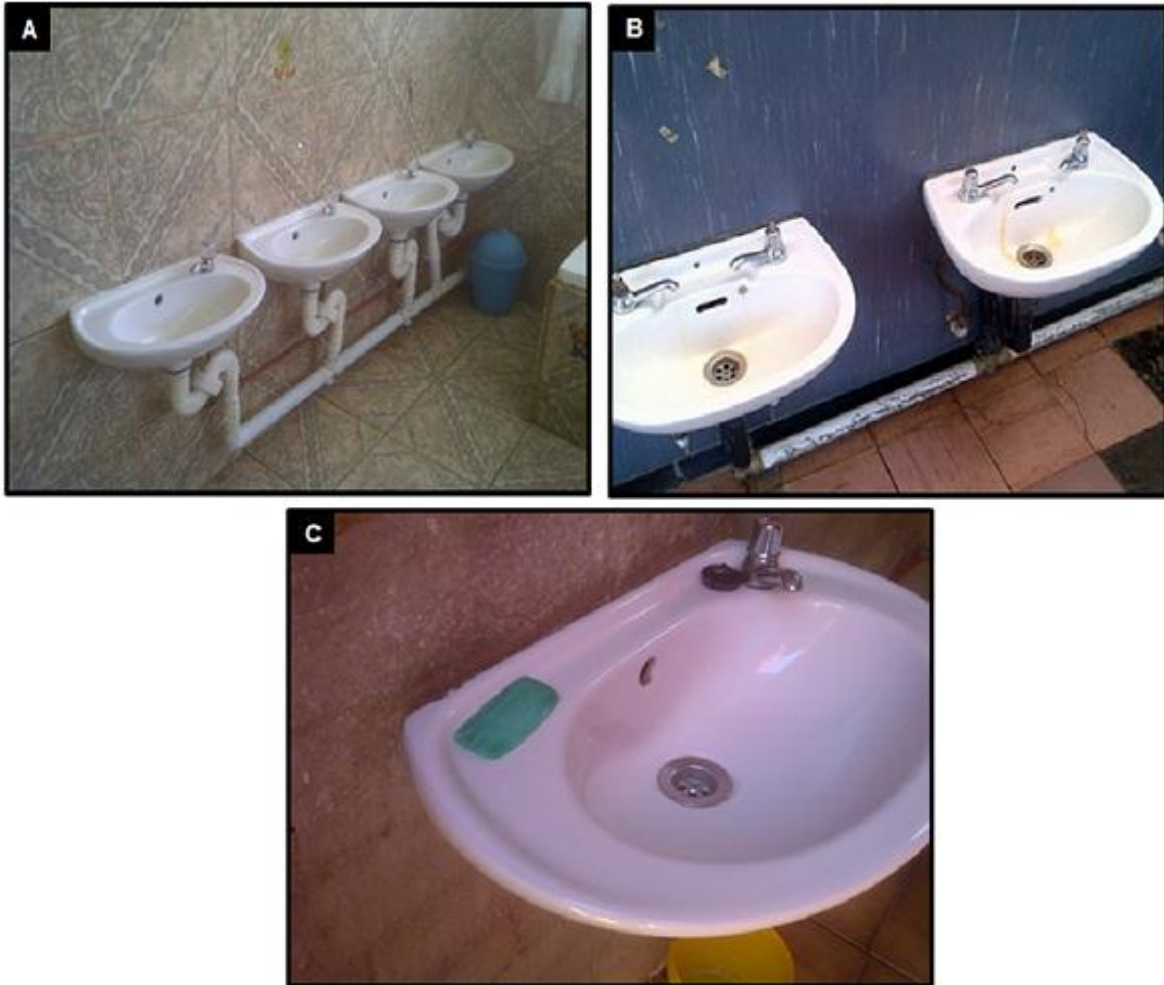
Figure 2.12: A-C Hand-wash basins. A- Wall mounted hand-wash basin; B- Wall mounted hand-wash basin with dismantled taps; C- Wall mounted hand-wash basin with hand-wash soap.
