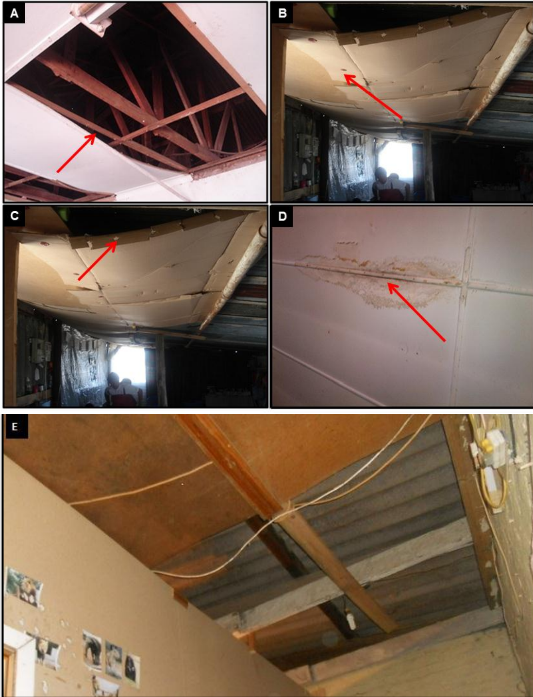
Figure 2.6: A-D Structural defects identified in childcare facilities. A- Peeling paint from wall; B- Holes in zinc sheeting wall; C- woven polypropylene bag used to line zinc sheeting wall; D- Holes in zinc sheeting wall.
