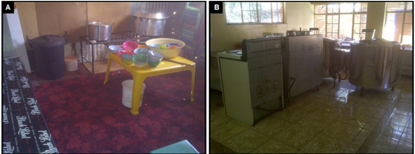
Figure 2.7: A-B Food preparation areas. A- Carpet floors in kitchen; B- Compliant kitchen with impermeable floors and waterproof walls.
