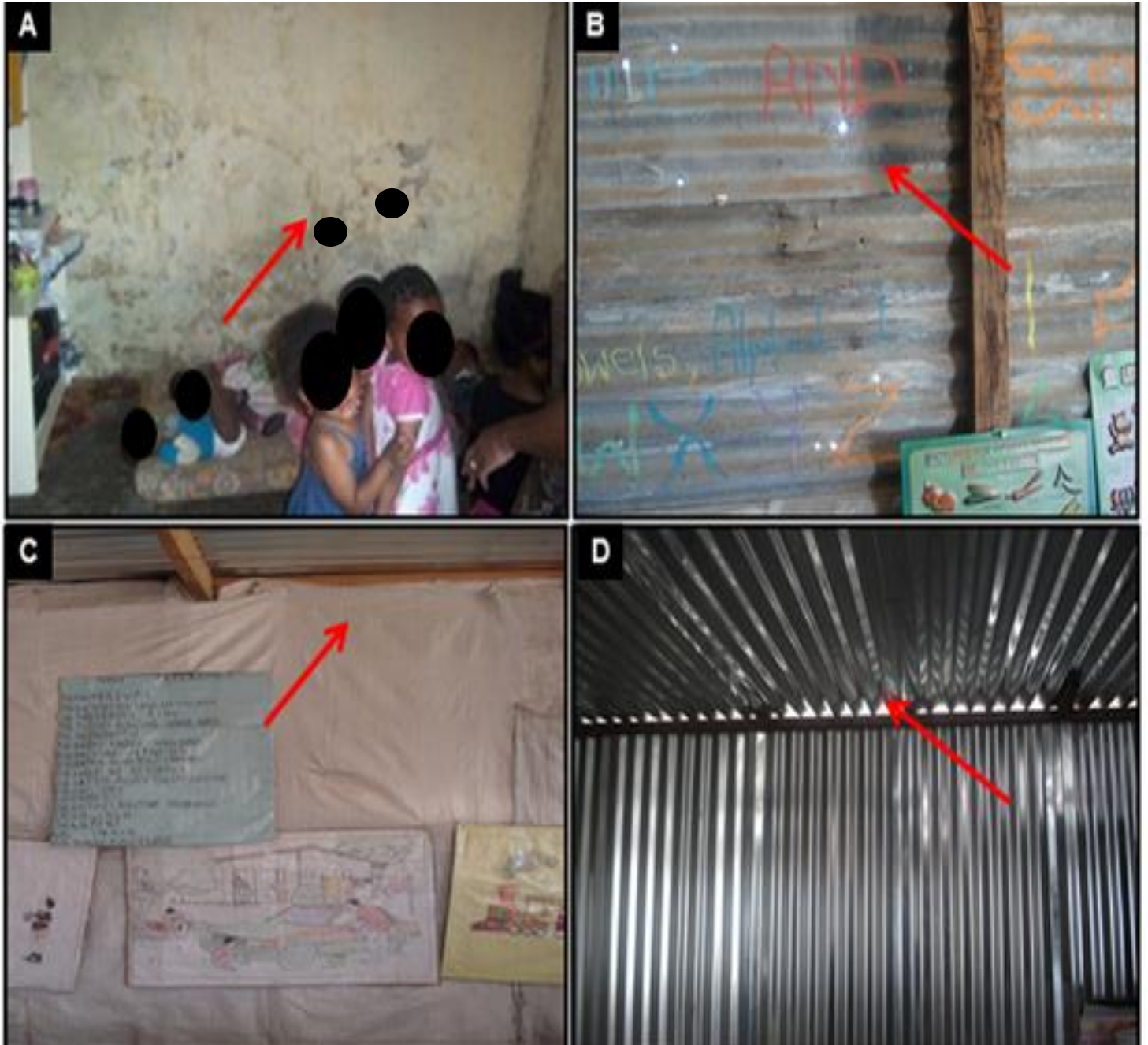
Figure 2.5: A-D Structural defects identified in childcare facilities. A- Peeling paint from wall; B- Holes in zinc sheeting wall; C- woven polypropylene bag used to line zinc sheeting wall; D- Holes in zinc sheeting wall.
