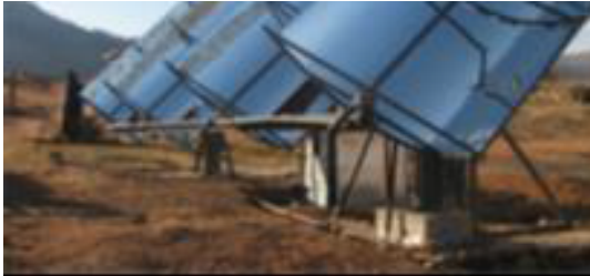
Figure 4.2 Parabolic reflectors (photo taken at Lesotho plant in the Berea district).
