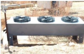
Figure 2.5 Air condenser side view with the three air fans at the top.
