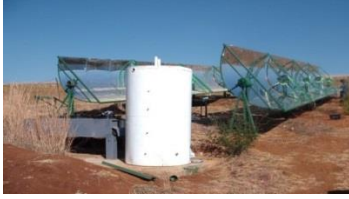
Figure 2.3 Photo of the white solar-thermal storage tank.
