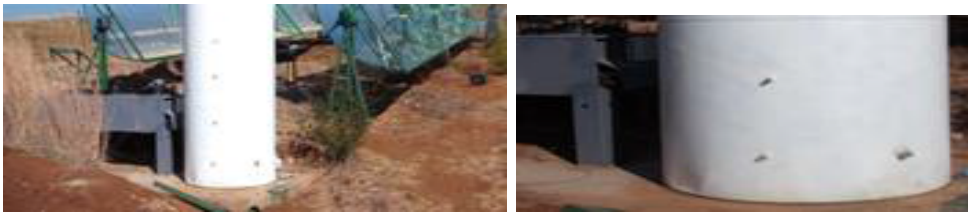
Figure 4.5 Photo of the thermal storage unit (white cylindrical tank)
