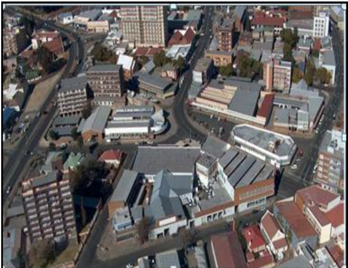
Figure 3.14: Aerial photo of the CBD of Kimberley City (Source: www.google.com Google earth, 2015)
