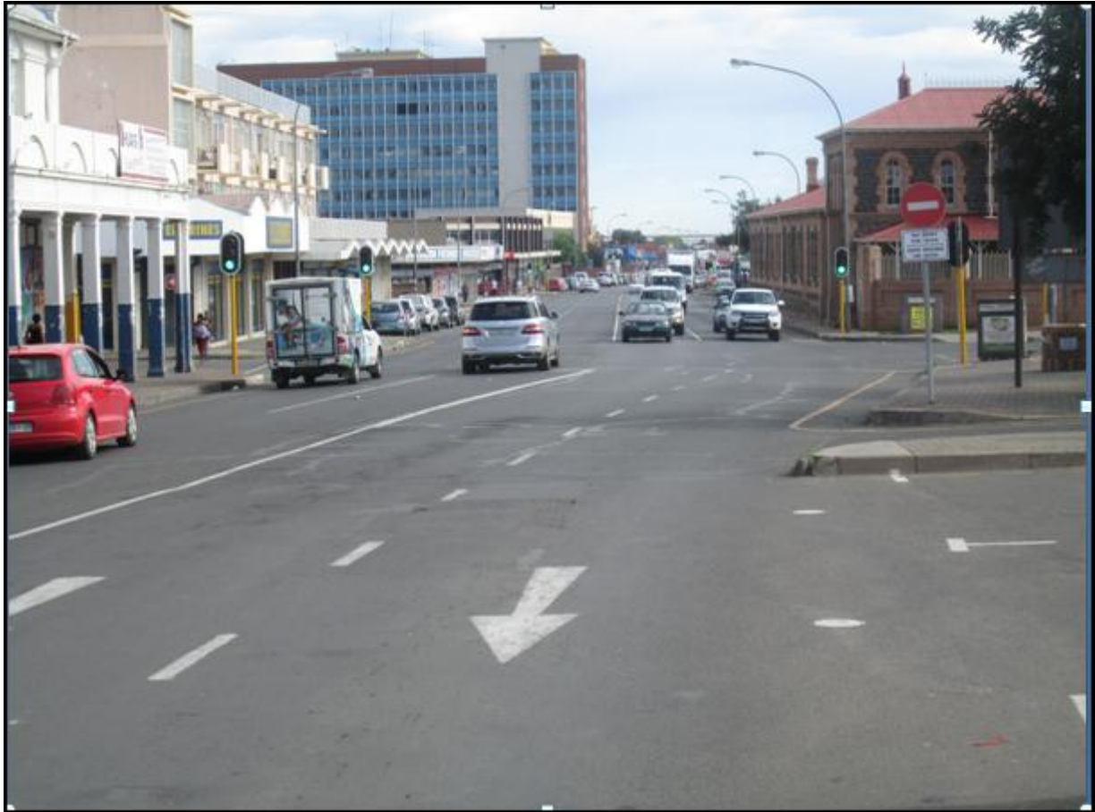
Figure 3.21: Traffic control facilities (pavement marking and lane demarcation) at the junctions in the Kimberley CBD area
