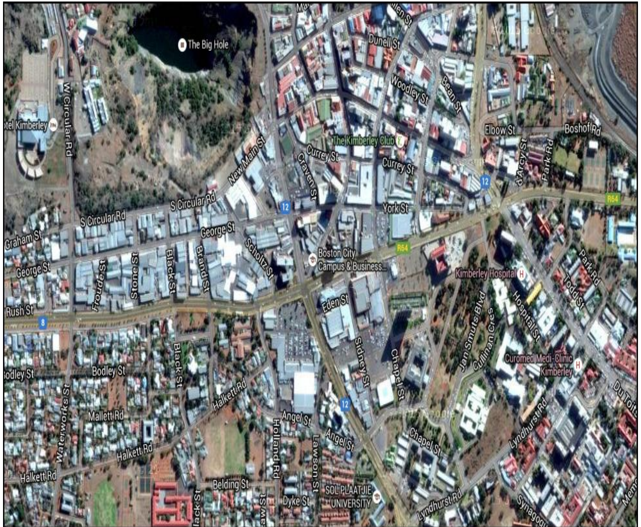
Figure 3.17: Internal road network of the Kimberley CBD area (Source: www.google maps.com, 2015)
