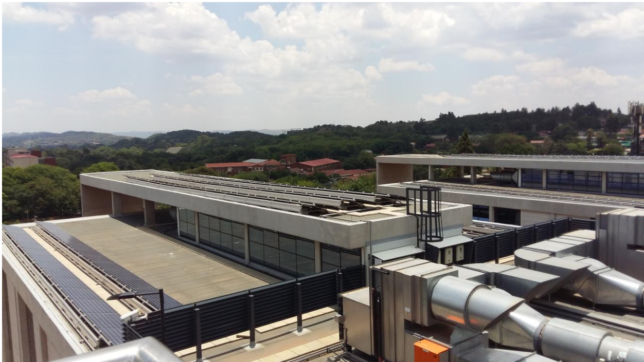
Figure 5.1: Central HVAC system fitted with automatic climate control system
