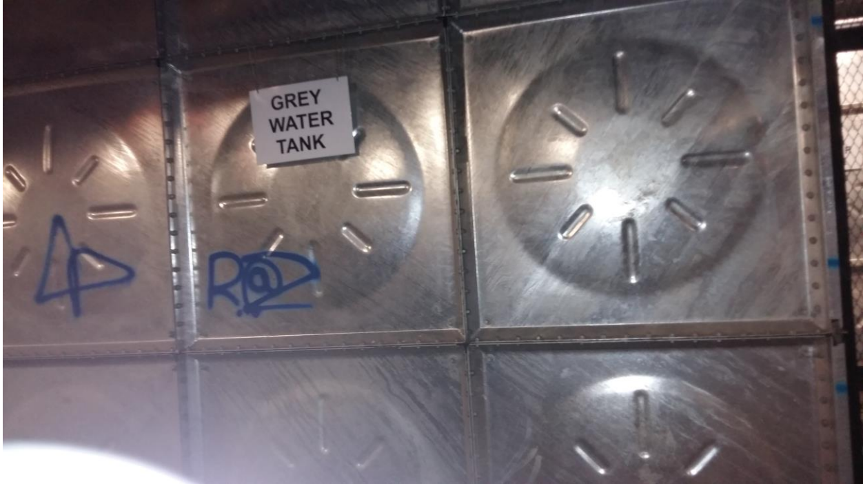
Figure 5.2: Underground grey water tank for water recycling
