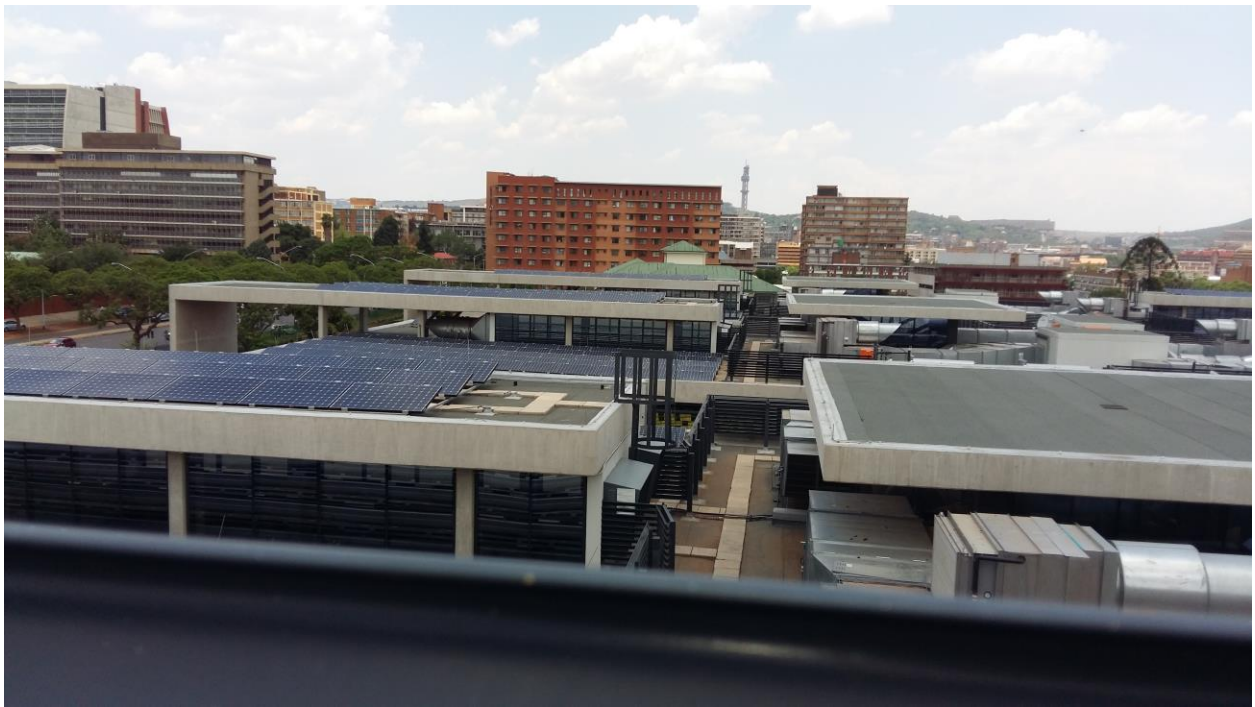
Figure 5.2: Arrangement of Photovoltaic solar panel for alternative power source
