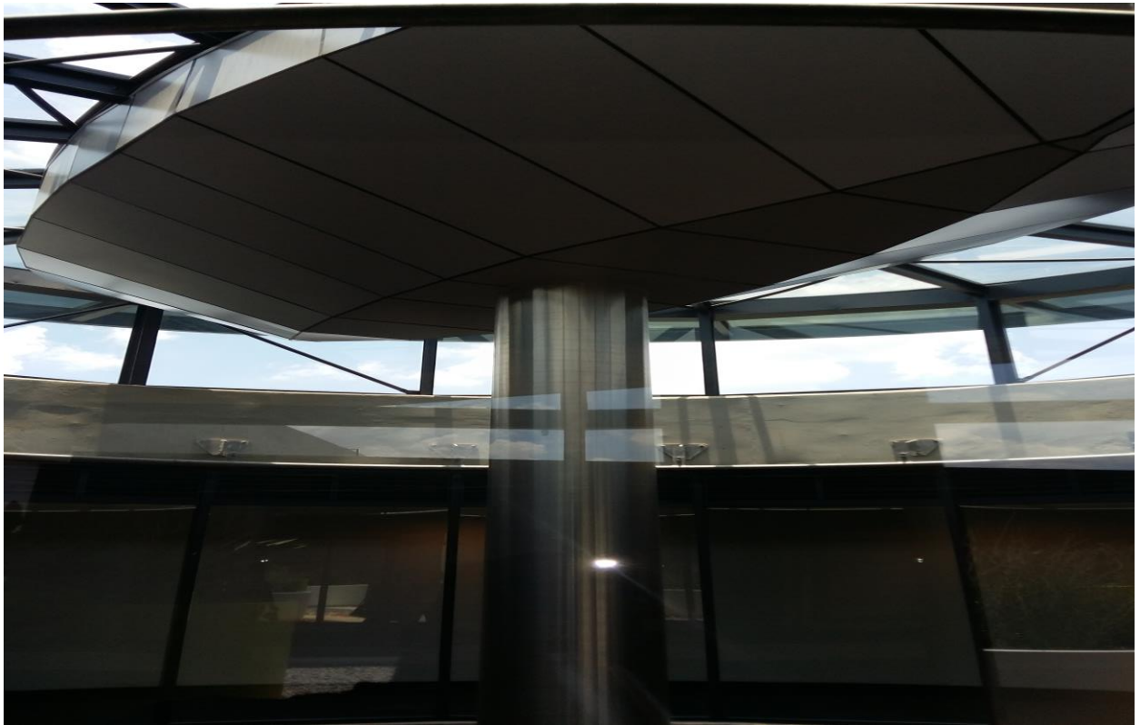
Figure 5.1: Rain-water harvesting dome for water management
