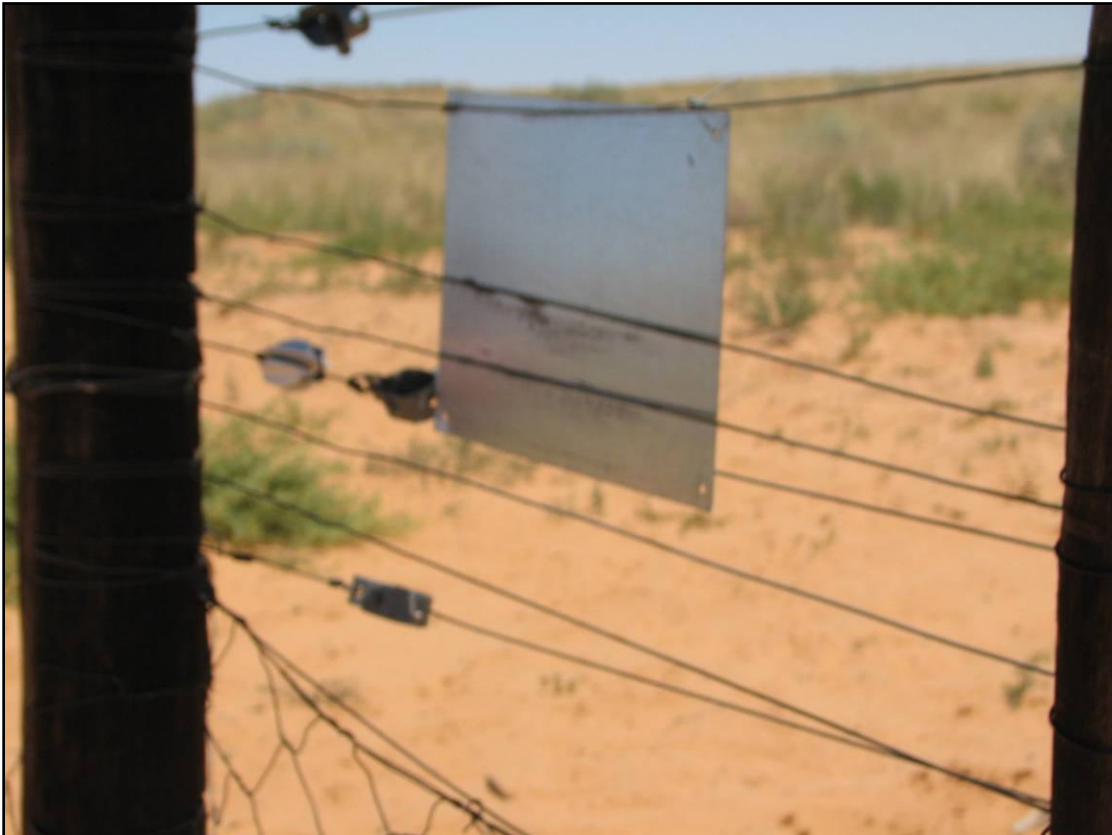
Figure 6.5 A flat metal sheet, fastened to both the KTP electric fence and the main fence, causes a short-circuit resulting in damage to energisers
