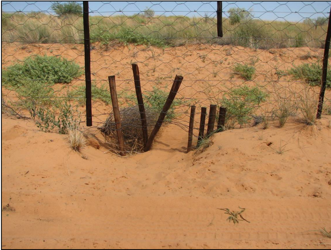
Figure 6.6 A burrow underneath the KTP fence. It had been covered with slats, but these had been pushed aside by either aardvark or porcupine. Such burrows are large enough to let predators, including lions, through.
