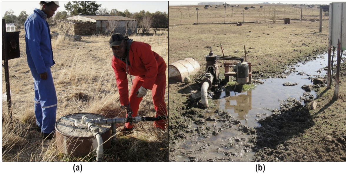
Figure 7.3 Borehole protection: (a) protected borehole head; (b) borehole head not elevated and not protected from stagnant water
