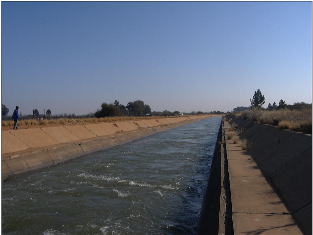
Plate 4.1: Combined trapezoidal canal (north canal)
