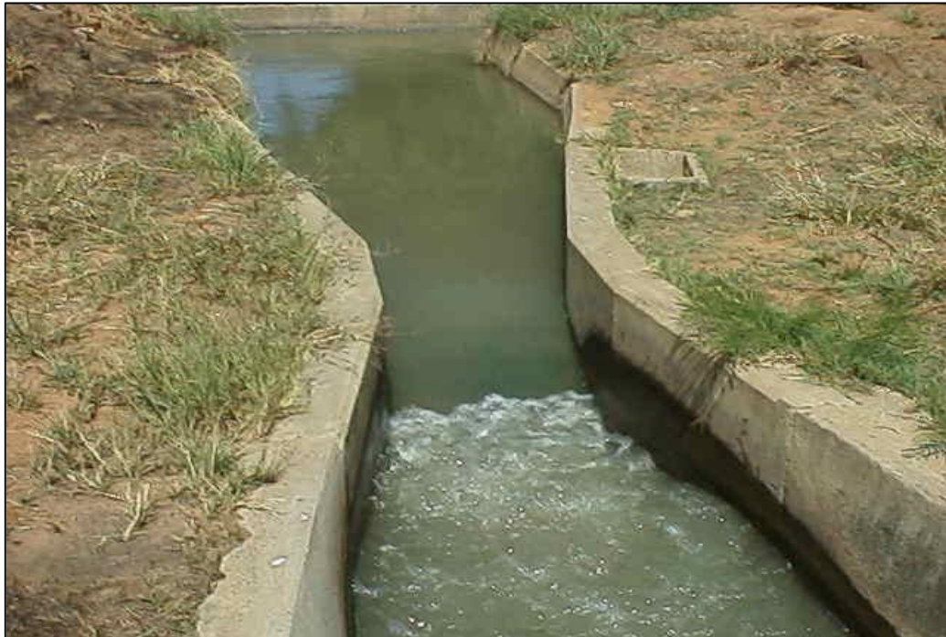
Plate 5.1: Parshall flume in Feeder 4
